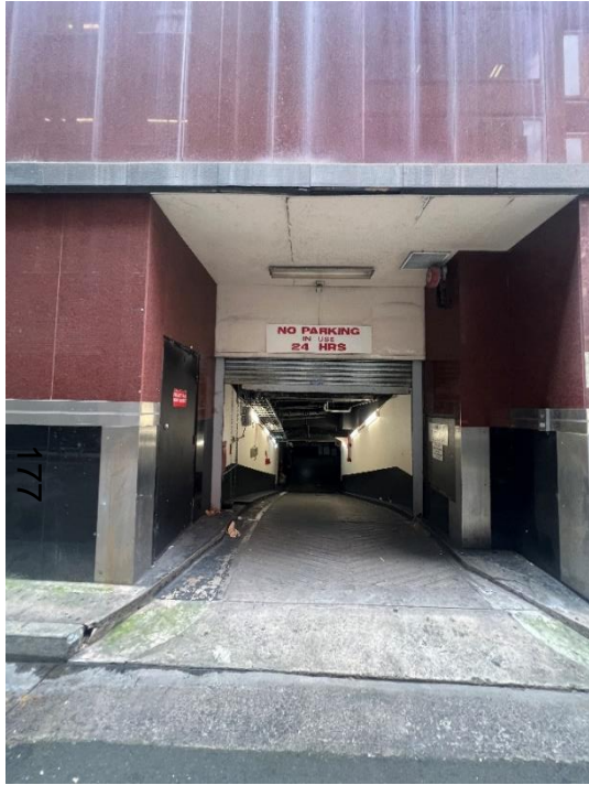
vehicle access from York Lane
